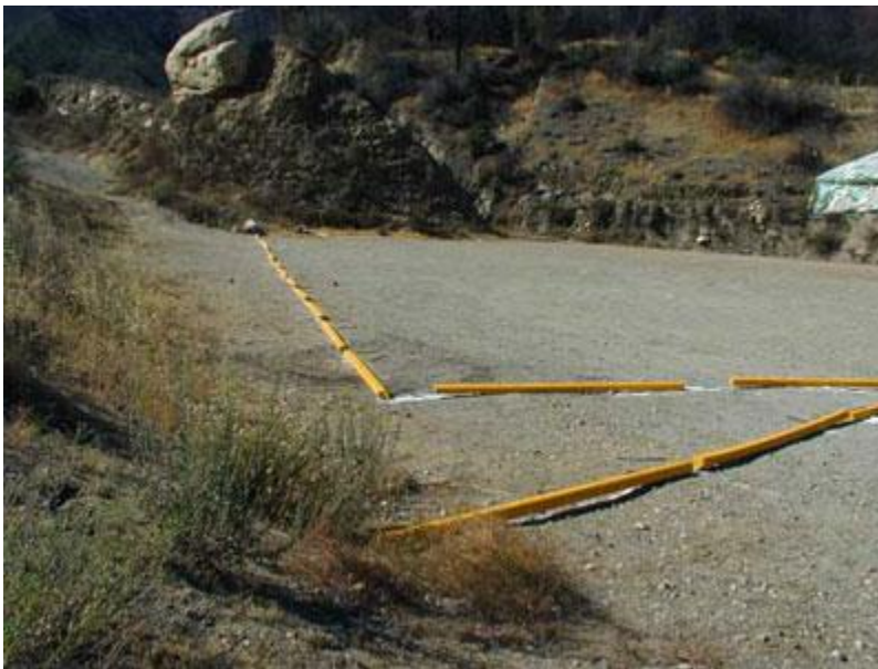
Figure 4.1.2: Wooden Delineators After Installation [Fed.US, 2016]
