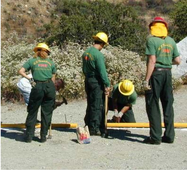
Figure 4.1.1: Installation of Wooden Delineators [Fed.US, 2016]
